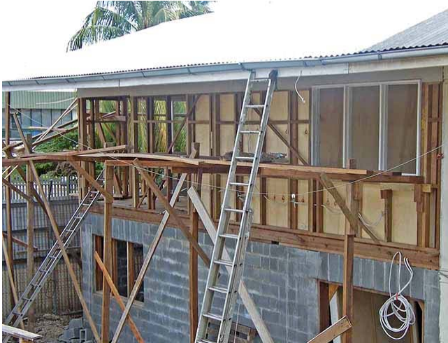
Oct. 4 Upstairs walls are started
