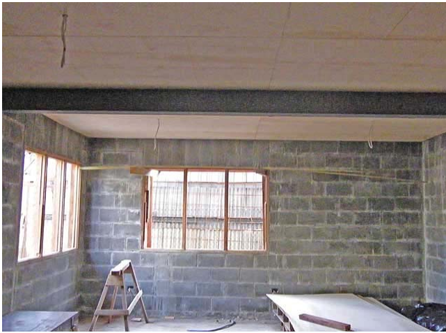
Oct. 4 Downstairs ceiling and wiring in place
