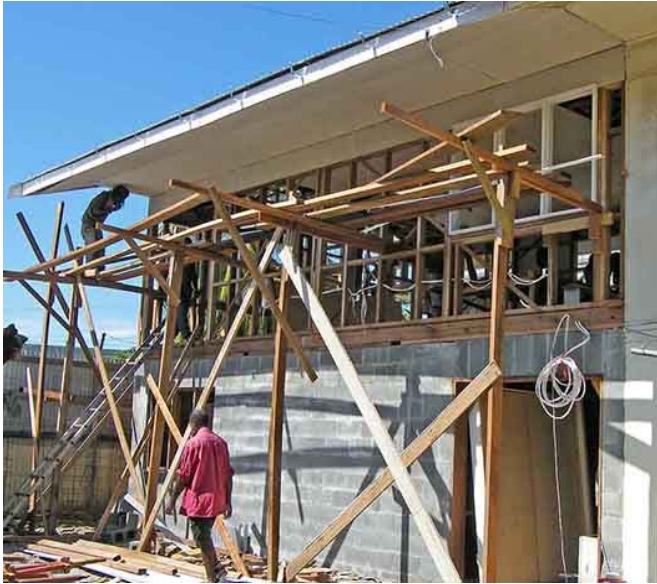
Oct. 3 The building is covered
