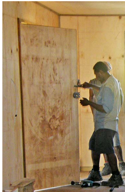
Oct. 10 And the doorknobs in place
