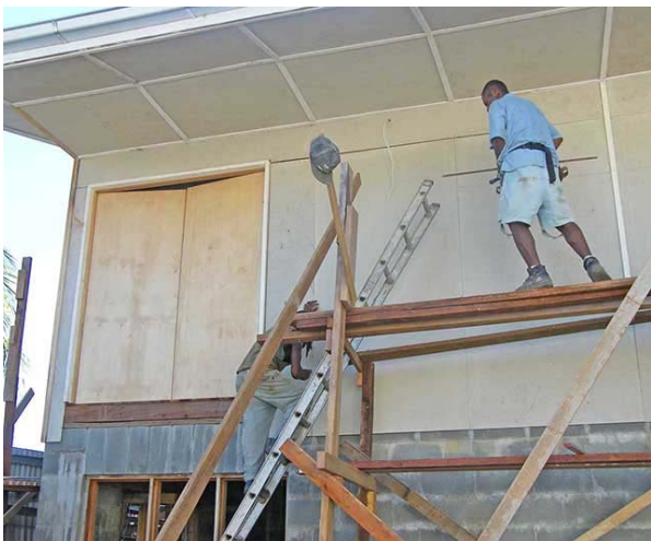
Oct. 7 The walls are up and doors are in!
