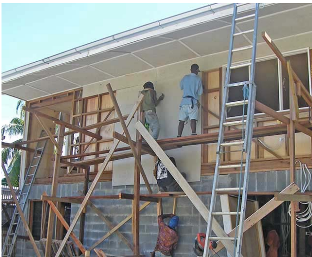
Oct. 7 Upstairs outside walls
