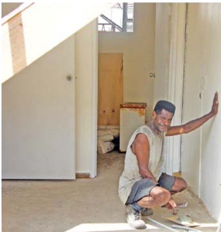
Oct. 16 First floor hallway & bathroom painted
