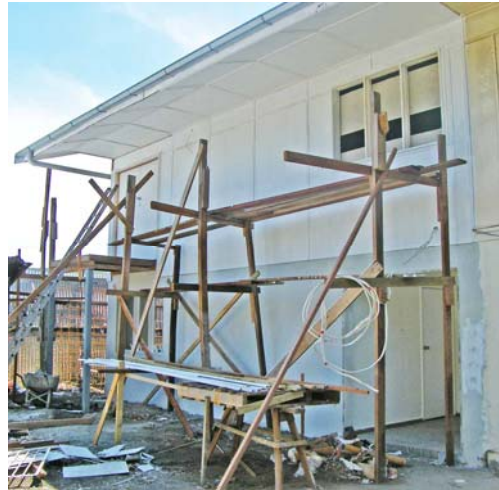
Oct. 18 First floor is stuccoed
