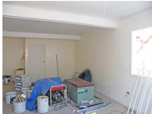
Oct. 18 First floor, second coat of paint
