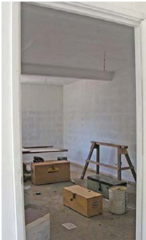
Oct. 13 First floor, first coat of paint
