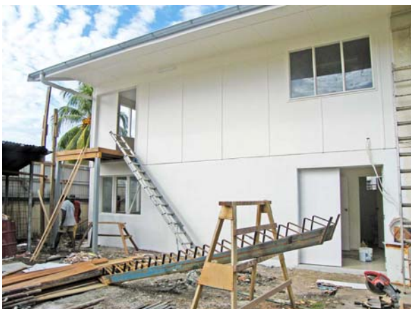
Oct. 25 Second coat paint; stairs awaiting!
