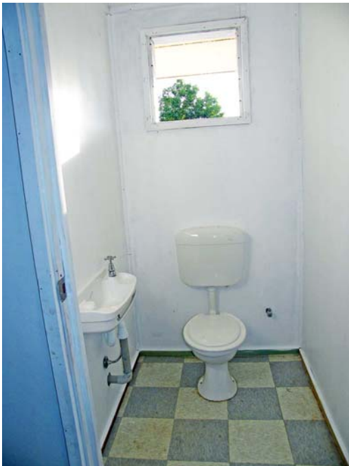
Oct. 21 Plumbing in the bathrooms
