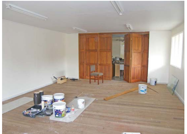
Oct. 25 Second floor, second coat of paint and lights
