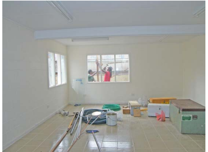
Oct. 25 First floor, Tile floor and lights
