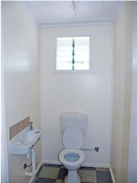
Nov. 1 Bathrooms are completed!
