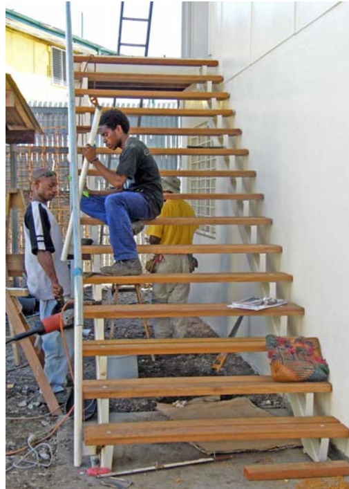
Nov. 3 Outside stairs up, railing almost up!
