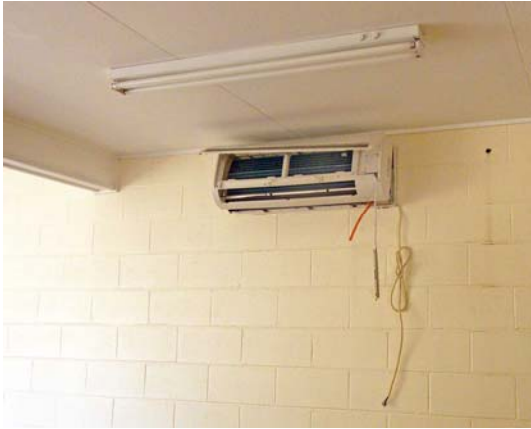
Oct. 31 Downstairs air conditioner still needs work
