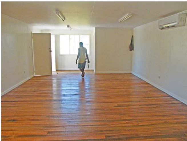
Nov. 3 Upstairs floor varnished, air con installed
