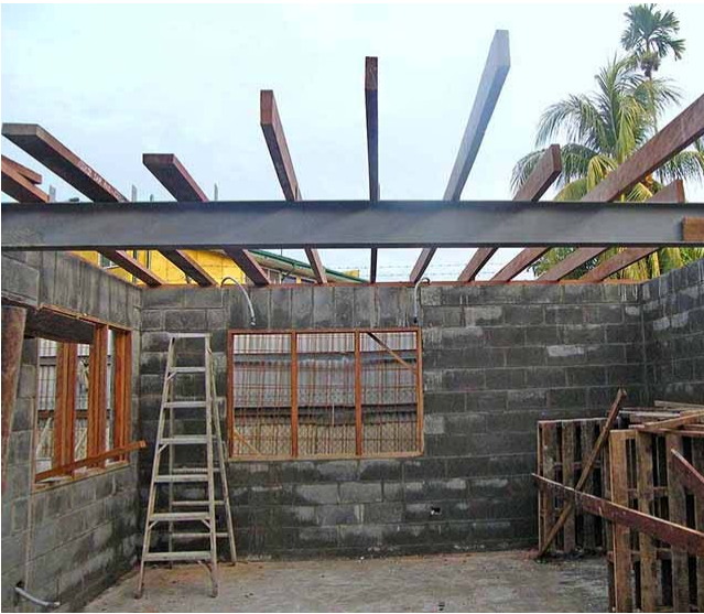
Sept. 18 Upper floor begins (taken from first floor)
