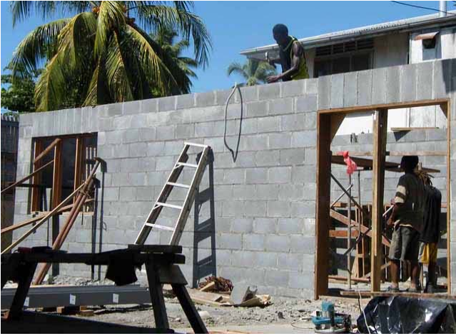
Sept. 16 Lower floor wall completed
