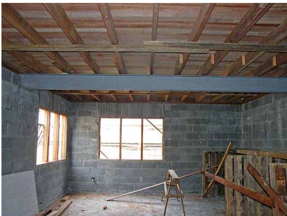
Sept. 22 Upstairs floor (taken from first floor)
