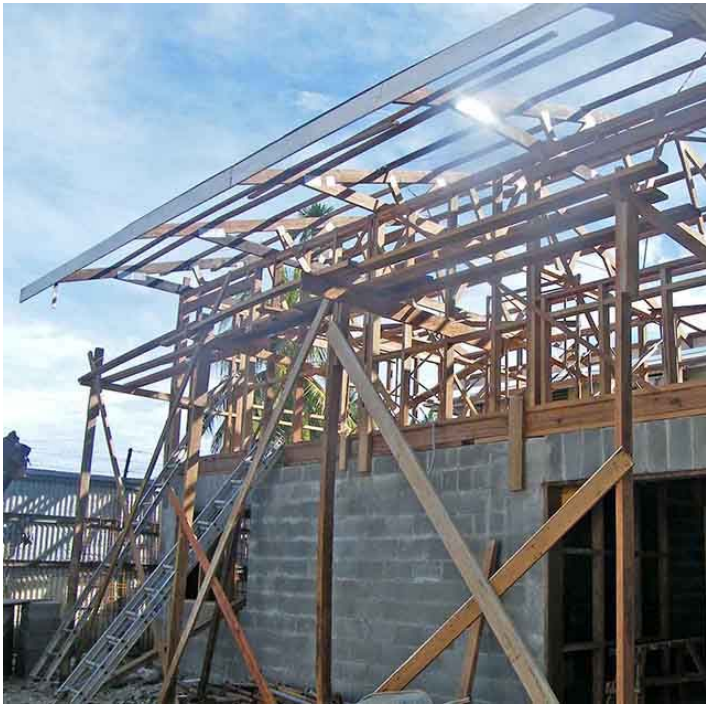
Sept. 30 Roof and upstairs walls continue to progress
