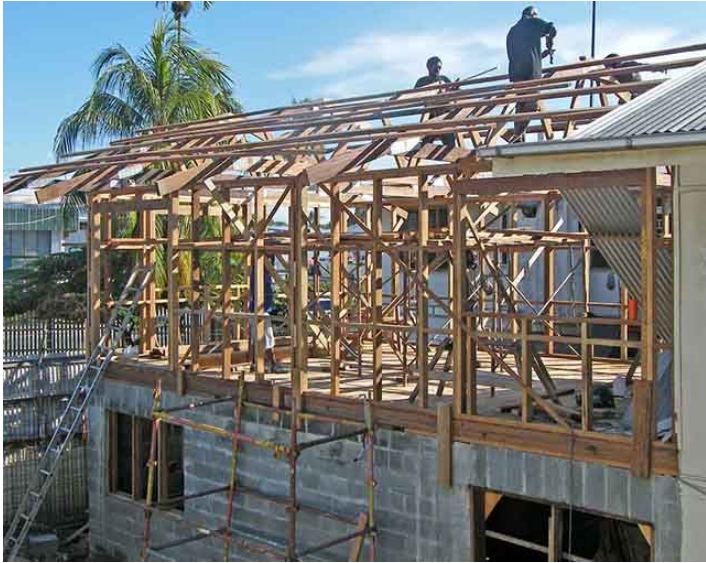
Sept. 27 They've begun the roof
