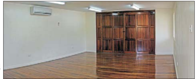
Pouring the slab, working on the second floor, and the completed multi-purpose room – only a few of the step-by-step pictures you can view at www.pioneerbible.org.pg .
