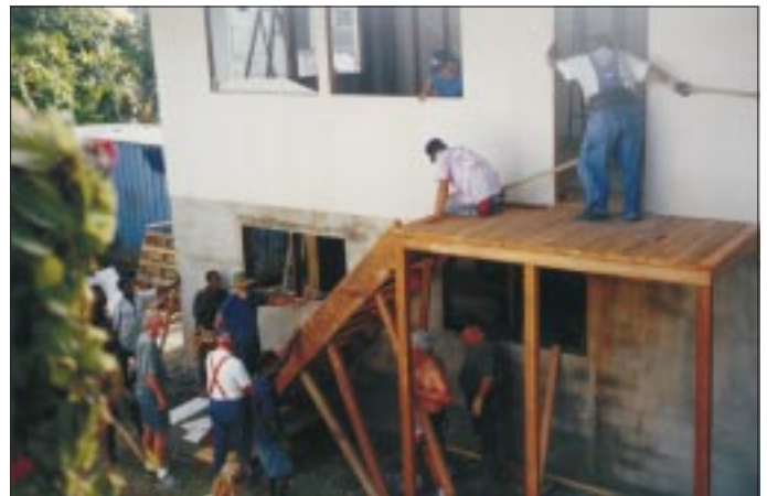
It took 10 men to place these heavy-duty kwila stairs.
