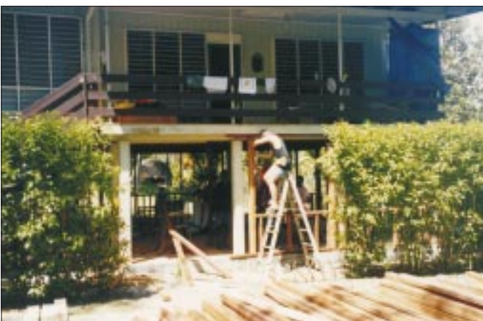
Rod Hildebrand sets another stud under the present Crescent House.
