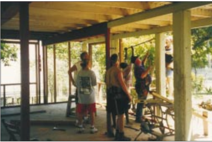
Framing under the Crescent House
